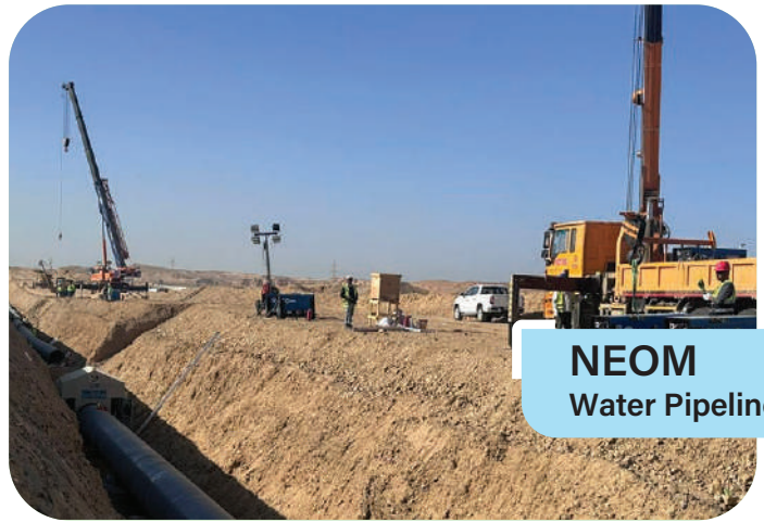
NEOM Water Pipeline
