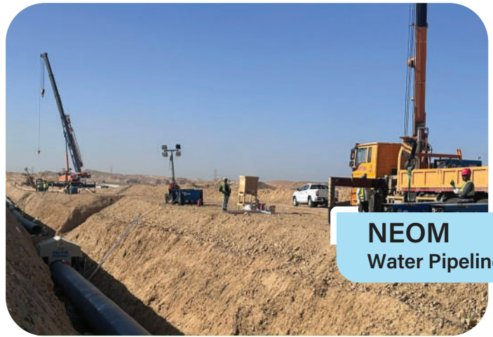
NEOM Water Pipeline
